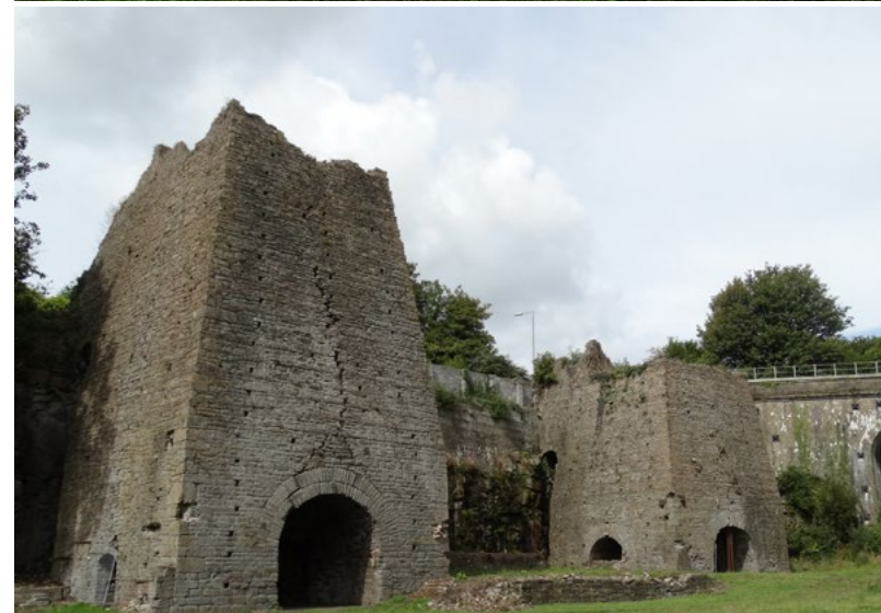
The work of dedicated volunteers who cleared vegetation from the Blast Furnaces at Neath Abbey Ironworks.
