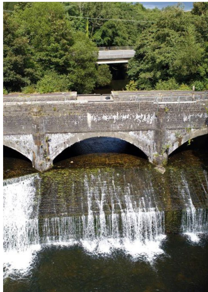
Canal Aqueduct over Afon Twrch, including weir, Ystalyfera (Grade II* Listed Building).
