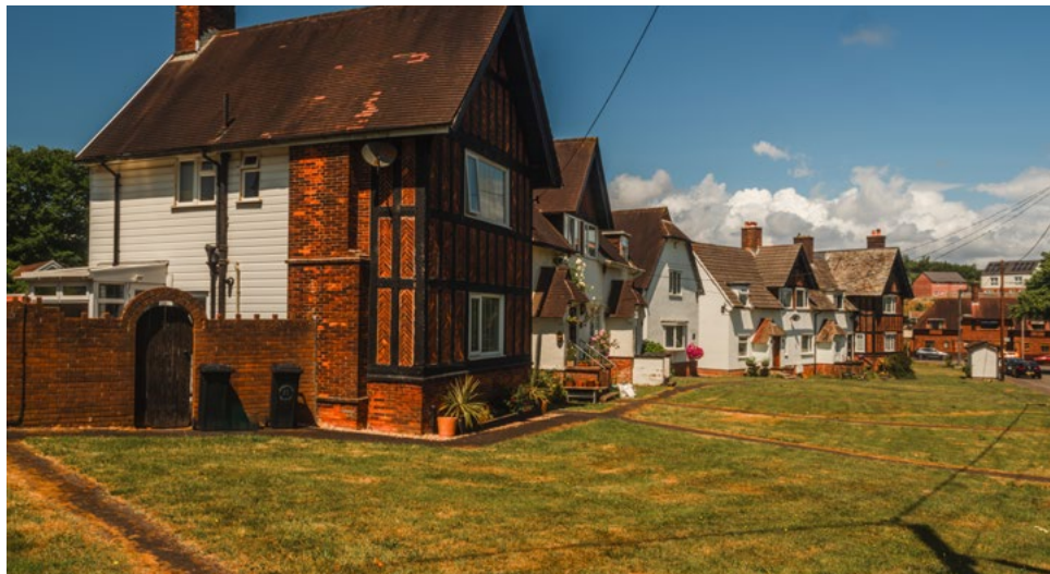
Unchecked adaptation to properties are diluting the appearance, character and special interest of our designated Conservation Areas. Llandarcy Conservation Area and Glynneath Woollen Mill Conservation Area.
